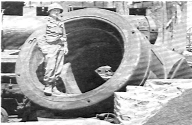
Breech ring, showing forward section. Note interrupted thread. Below: detail of blown-off section of forcing cone of tube No. 1.
